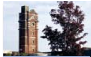
The striking Water Tower is a recognisable landmark visible for miles around.
