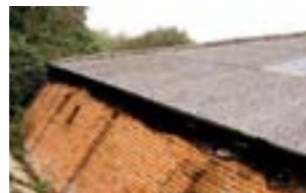
Grade II Listed 17th Century barn.
